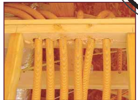
Kwikpath Resi is a convenient, flexible raceway system to meet the current and future cabling needs of any homeowner.
